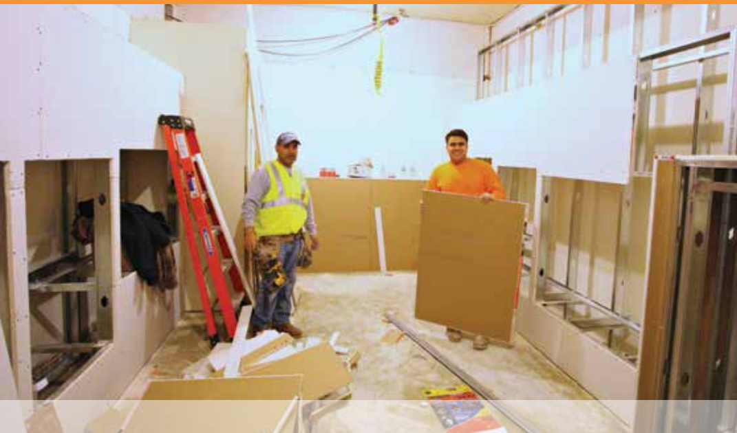
Construction begins on The Terrace's new mail room.
